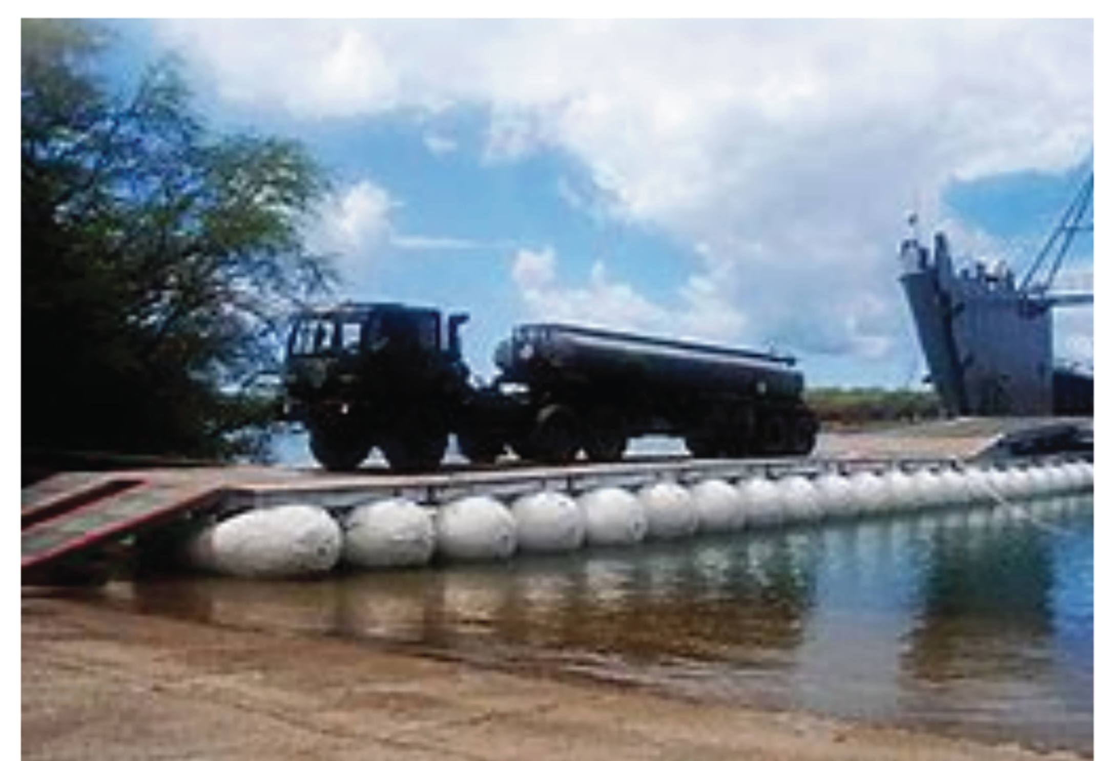
Figure 3: Trucks crossing modular floating bridge
